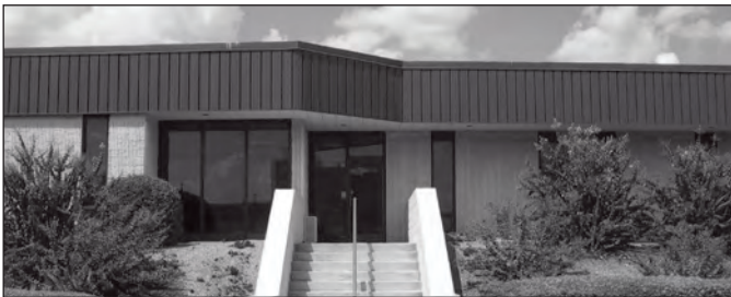
Olive Branch, Mississippi, USA Manufacturing and Distribution
