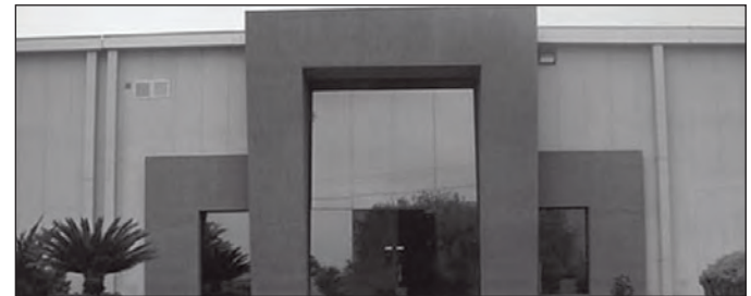
Monterrey, Mexico Manufacturing and Distribution
