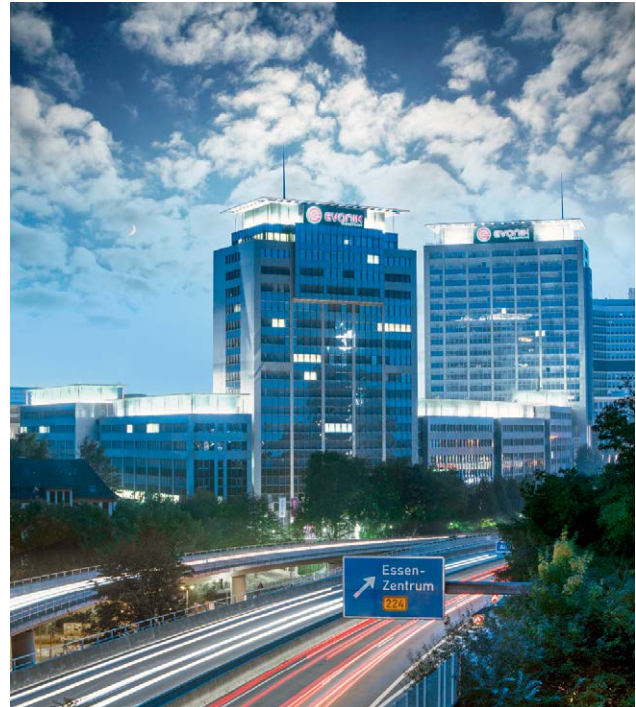
Evonik's company headquarters in Essen
