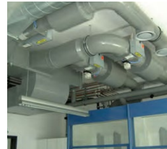
Fume vents, ducting: SIMONA® PVC Type I
