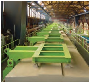
Plating and pickling tanks, covers: SIMONA® PP
